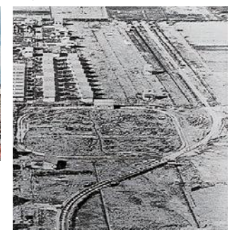
東苗穂自動車訓練所に造られた広大な地下鉄試験場。Higashi-Naeho Car Training Center where subway trains were tested.
