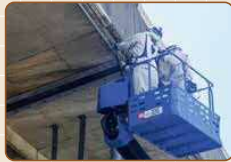
橋梁の目視点検
