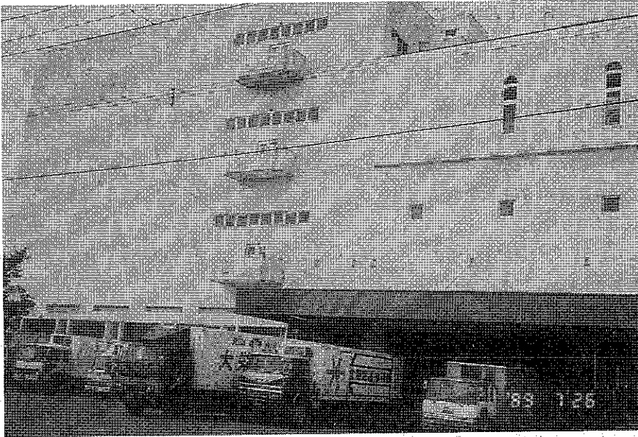
Fig. 6 Photograph of Deep Freeze and Cool-Storage Plant
